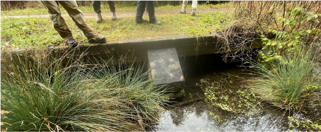
CulvertA_Concrete Box - Two culverts near the Hillsburgh Trailhead
