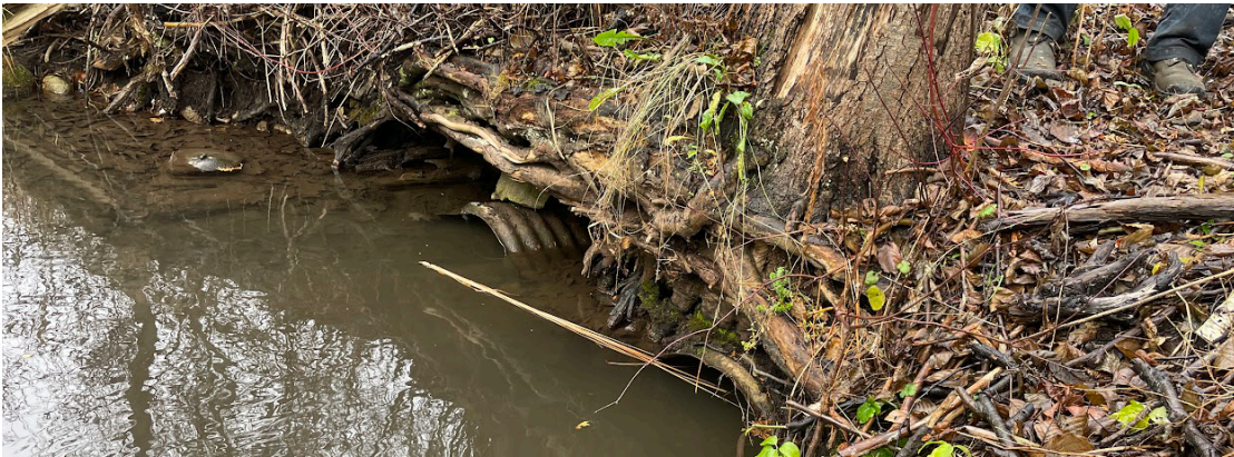
CulvertB_CSP - Two metal culverts near the Hillsburgh Trailhead
