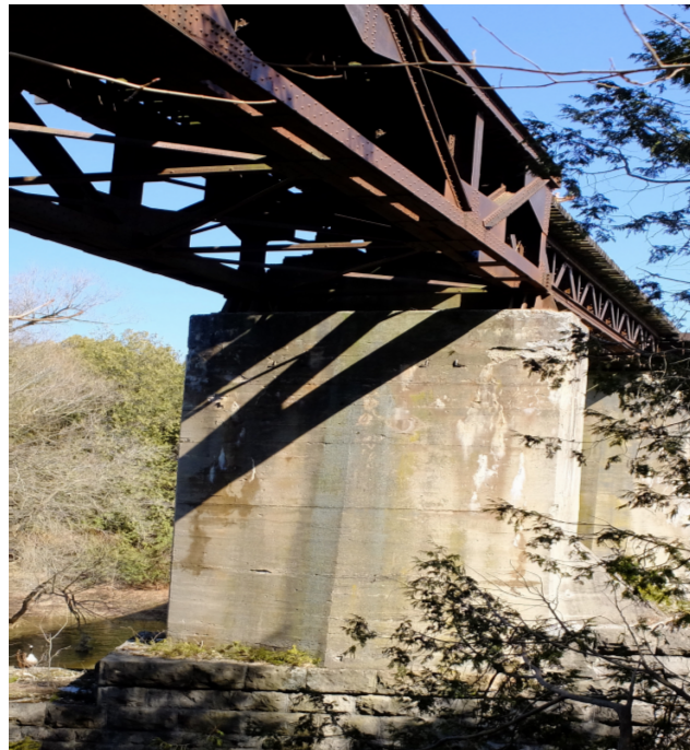
Trestle Bridge stone pier
